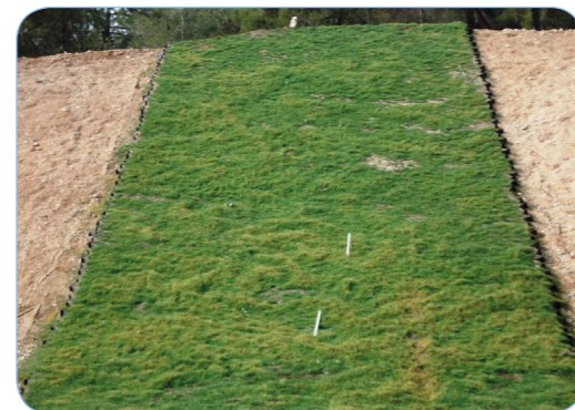
Embankments / Slope Protection
