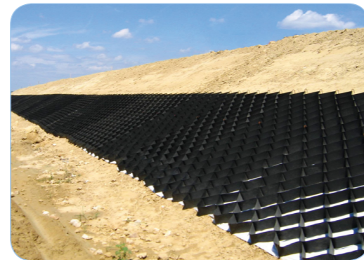
Embankments / Slope Protection
