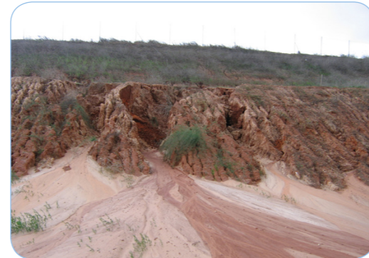
Embankments / Slope Protection
